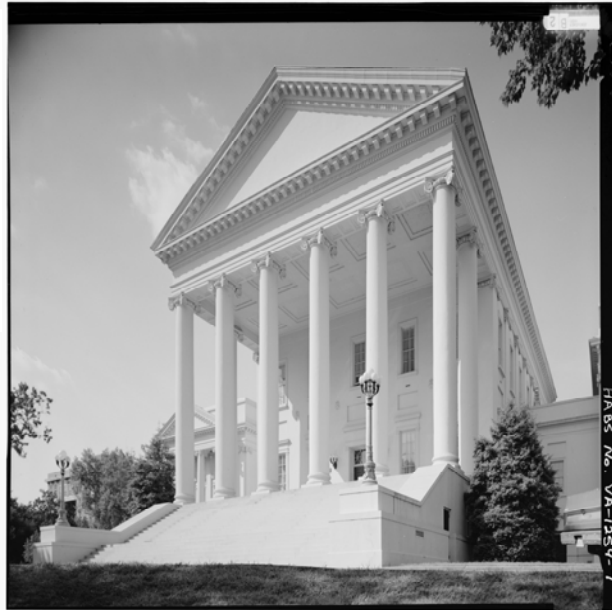
Figure 3. Virginia State Capitol, Richmond Virginia, Southwest Facade. Reproduced courtesy of Library of Congress, Prints and Photographs Division, Historic American Buildings Survey.
