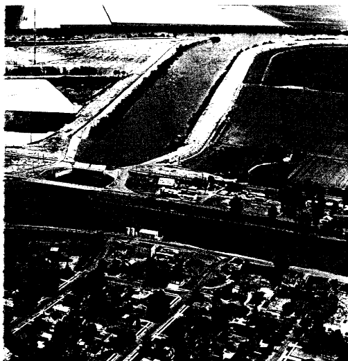
The Delta Cross Channel near Walnut Grove, part of the CVP, carries Sacramento River water south and west to the export pumps near Tracy.
